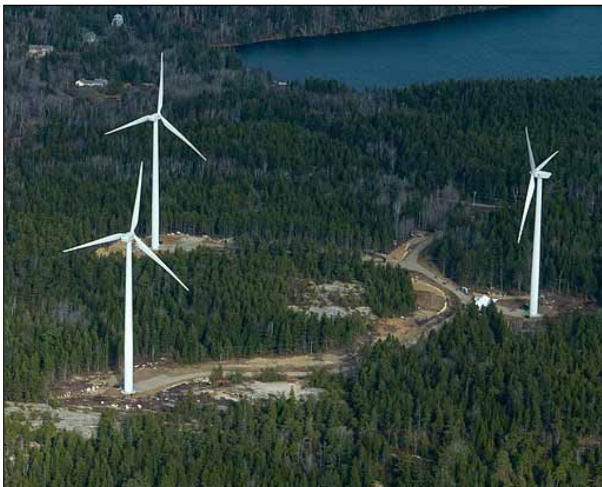
Wind turbines on Vinalhaven.
